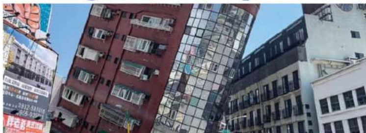
In this image taken from a video footage run by TVBS, a partially collapsed building is seen in Hualien, eastern Taiwan on April 3, 2024. An earthquake rocked the island, collapsing buildings in a southern city and creating a tsunami that hit southern Japanese islands.
