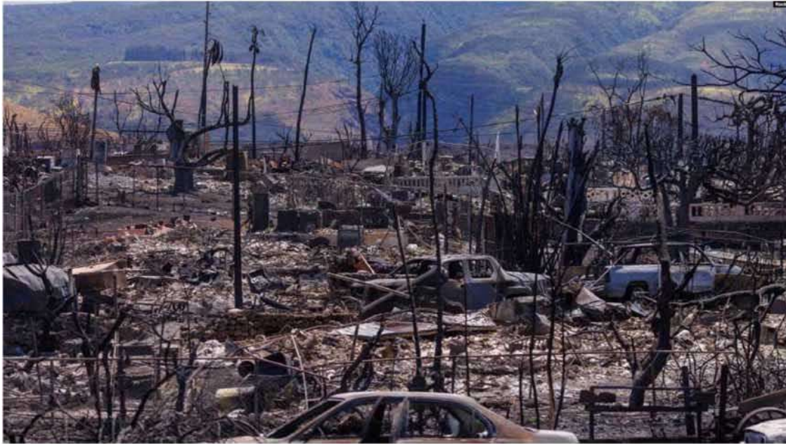
Fire damage is shown in Lahaina, Maui
