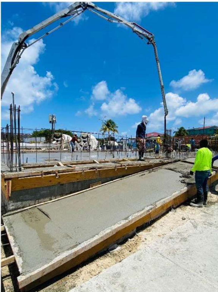
Highlights from the 18th April, 2023 concrete pour of the ground floor.
