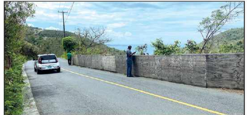
Area for the upcoming road rehabilitation and slope stabilisation works
